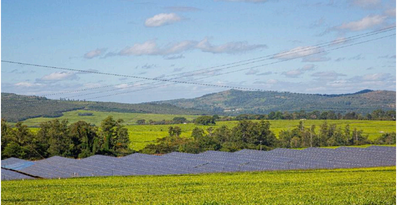
Solar plant at Ratelsboek estate
