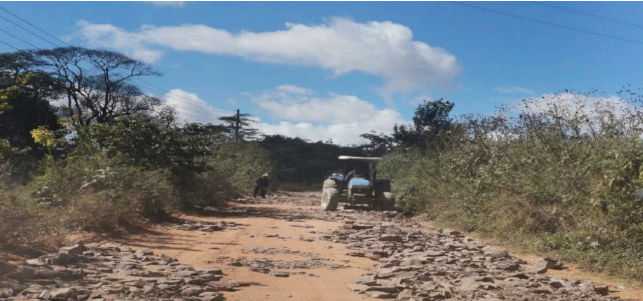
Community road repair
